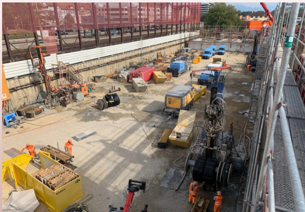
Figure 4.11: Well services teams prepare to drill a series of shallow geothermal boreholes to provide commercial-scale heating and cooling in the urban area of Lausanne, Switzerland. Photo courtesy of Groupe Grisoni.
