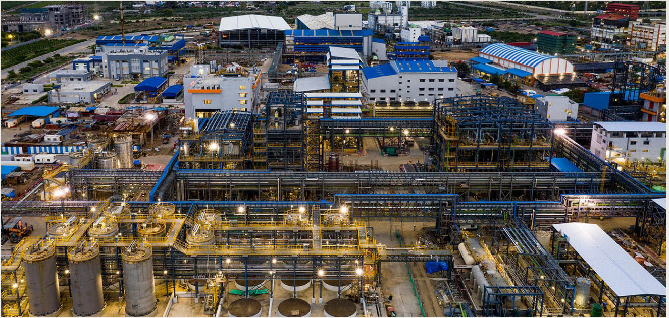
Figure 3.4: Aarti Industries industrial facility in Jhagadia, Gujarat. Source: Aarti Industries.
